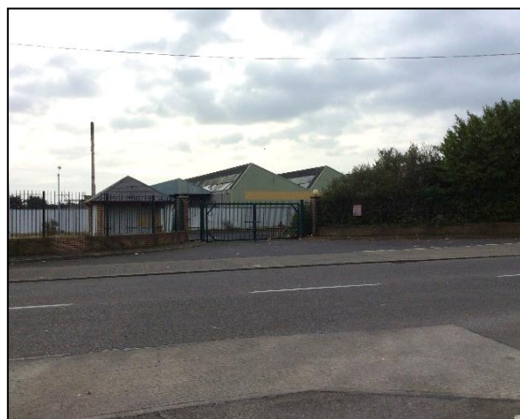
EXISTING ACCESS OFF COOLOCK DRIVE
