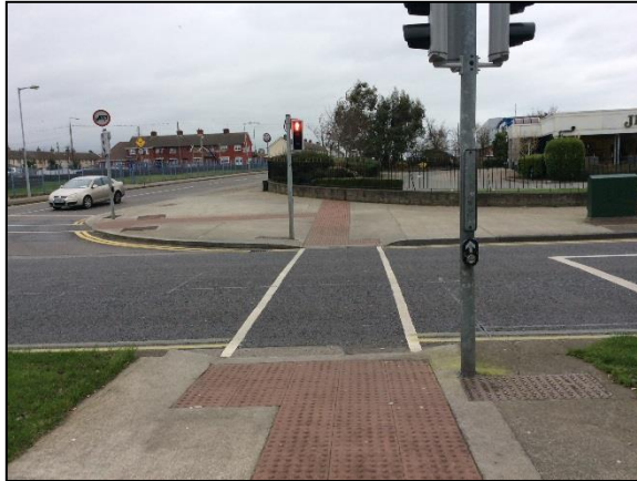
FIGURE 6.4 EXISTING PEDESTRIAN CROSSING ON OSCAR TRAYNOR ROAD
